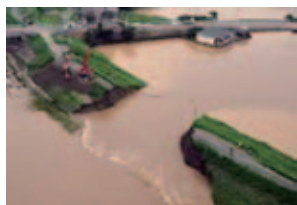
Levee breach by piping
