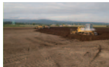
Construction of large-sized paddy field: Decision on selection of machinery and construction timeframe based on the soil diagnosis is required.
