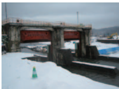
Example of deterioration of irrigation facilities: pier of the headworks with wear and frost damage, and gate with wear and corrosion
